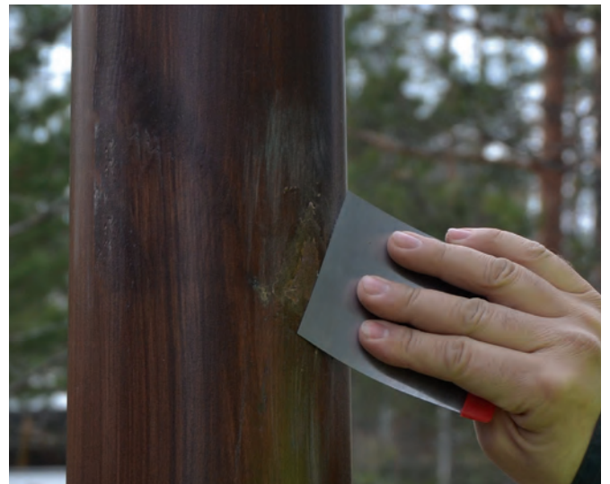
Applying epoxy
